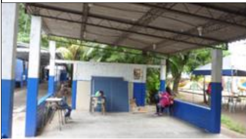
Vista general interna
