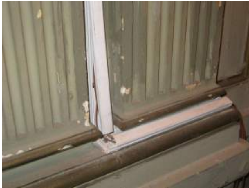
76-INSTALACION NO ORIGINAL
