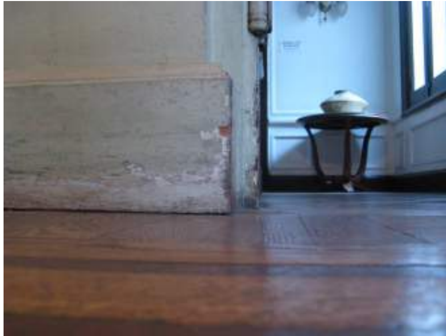
30-FALTANTE PARCIAL-PERDIDA DE RELIEVE-RAYADURA
