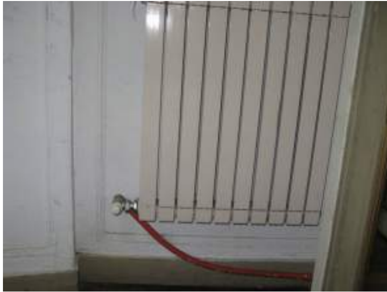
3-INSTALACION NO ORIGINAL-PERDIDA DE RELIEVE
