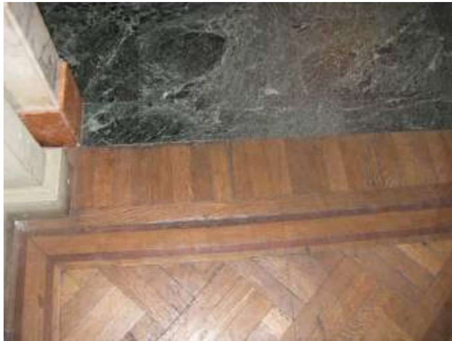
53-PI-DESNIVEL-SUCIEDAD SUPERFICIAL-RAYADURA
